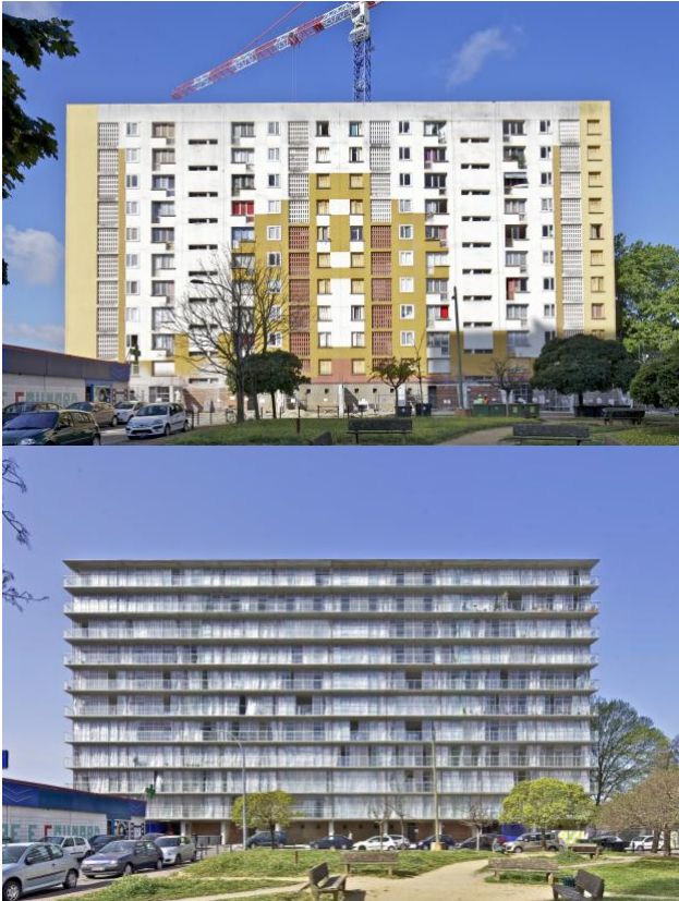
Before Retrofit (Top) and After (Bottom) Retrofit - Cité du Grand Parc, Bordeaux, France.
